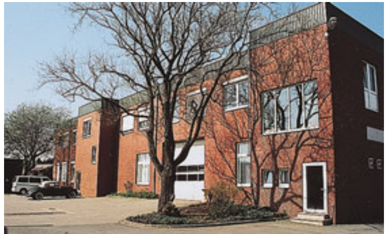
Training centre and R & D building
