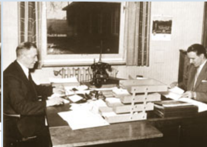
Part of the design office
