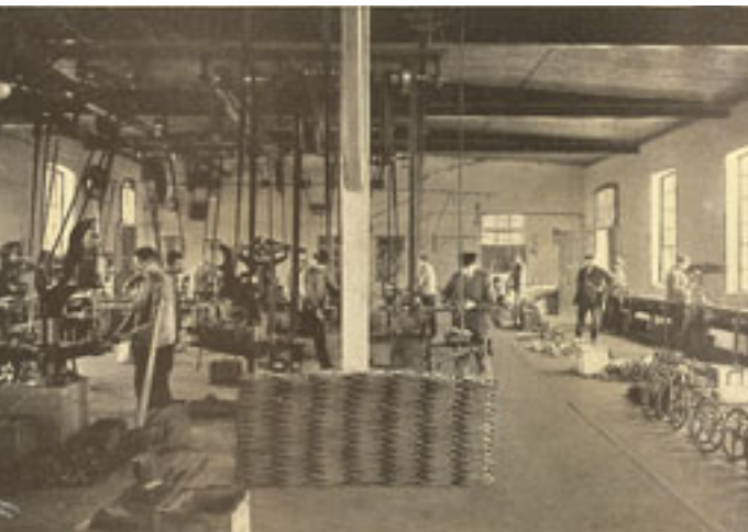
Lathes and drilling machines, driven by transmission shaft drive belts, 1912
