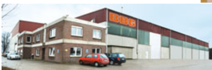
The site in Hude-Nordenholz for the production of our Cirrus large-area seed drills, 2004
