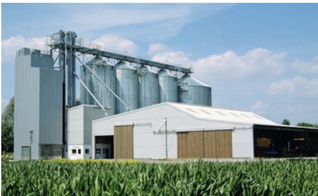
Bulk goods warehouse, 1971
