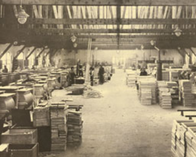
Large assembly hall, over 25 m self-supporting with nailed wooden trusses, 1912
