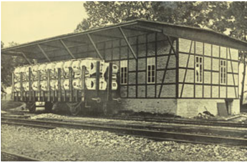
Storage and loading shed on the Osnabrück – Münster railway line in Hasbergen, ca. 1910. The machines were brought here by horse-drawn carts.
