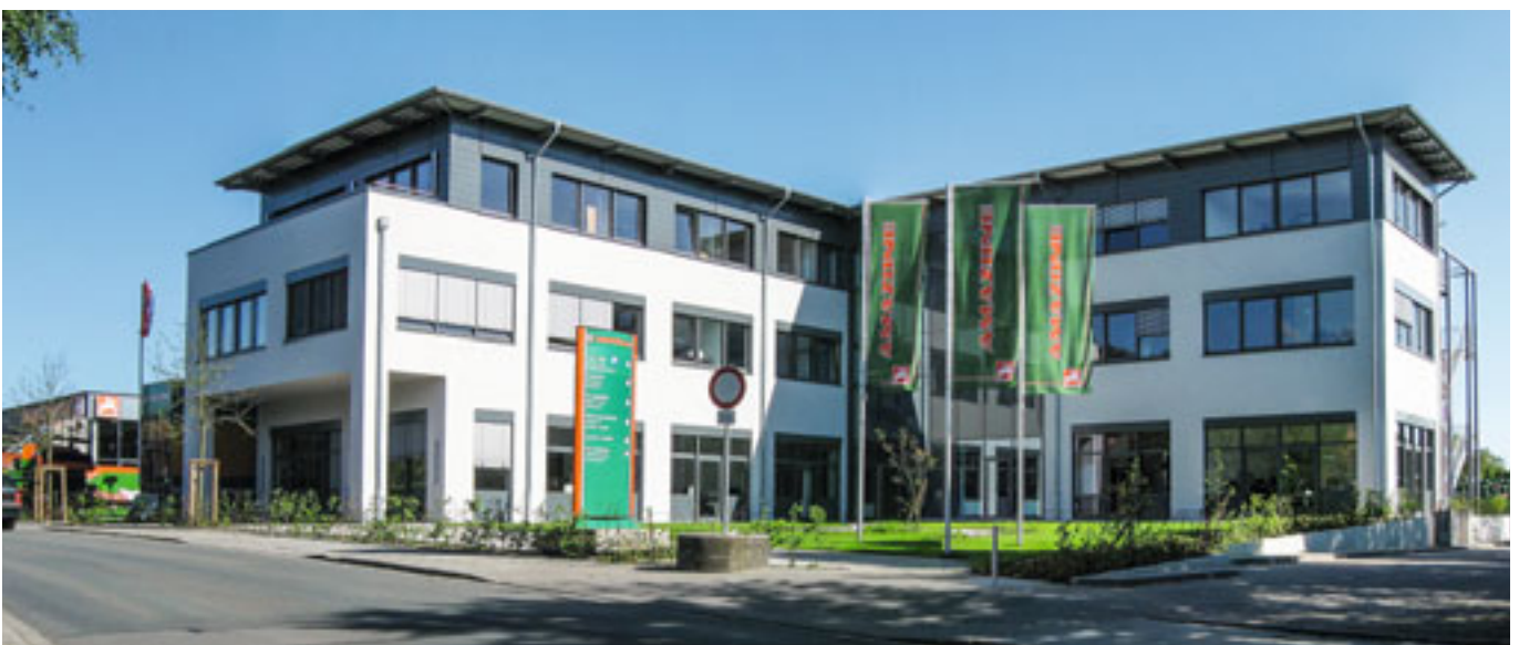
The new technology centre with 120 workstations in Hasbergen-Gaste, 2014
