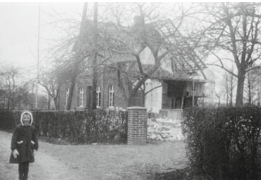
The badly damaged house of Johann Dreyer, in the summer of 1944
