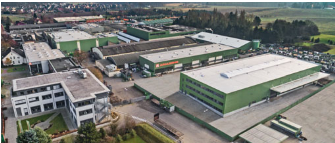
In Hasbergen-Gaste, the technology centre (left) and the test centre (right) now form a single unit.
