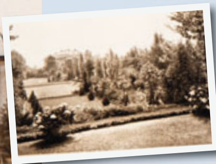
in 1905, a 25 ha park with a lake, flowerbeds and small pavilions was laid out at the experimental station.
