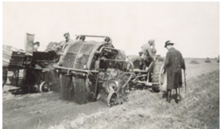
Potato harvester testing with basket collection wagon
